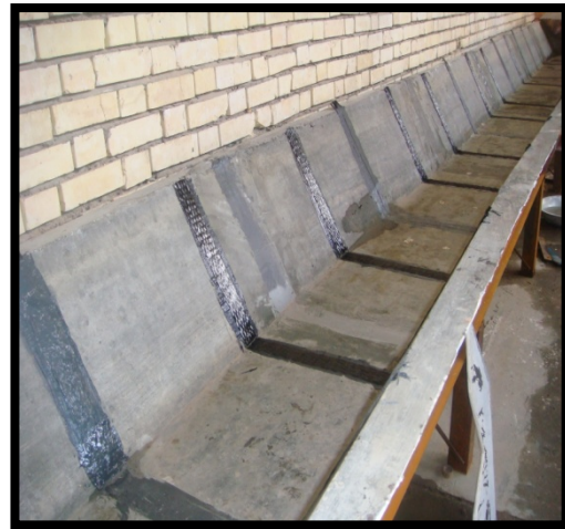
Photo 7 flume with 15 tapes from CFRP sheets
